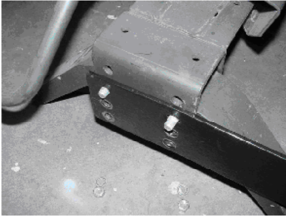
Figure 3-Left Side Plate installation
